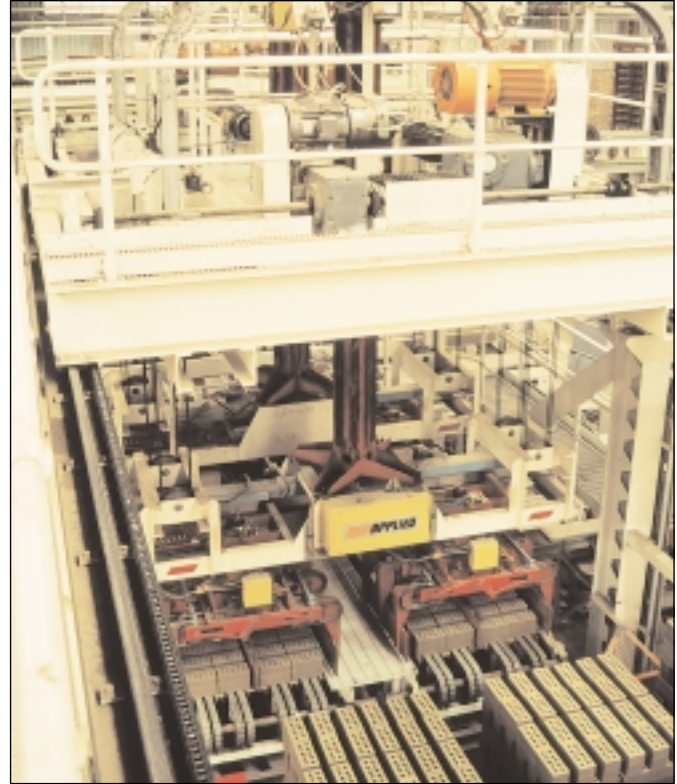
Baldor Vector Drives in a brick plant in Australia
